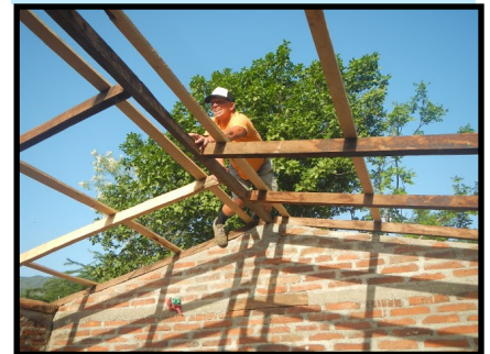
Replacing the church roof
